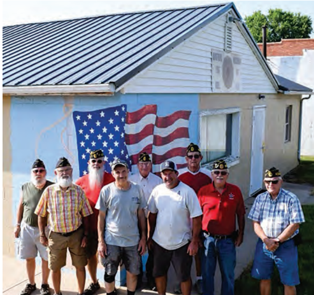
Odell Legion Post 231 would like to say THANK YOU to the Astro Bldg Company, Ed Zarybnicky, Ed Hajek & Matt Klecan for the material & labor to put the new steel roof on the Odell Legion Bldg! Pictured (L to R) Bill Shoff, Mike Riggert, Mark Billesbach, Ed Hajek, Duane Colgrove, Ed Zarybnicky, Commander Ron Wieters, Gary Bures, and Adjutant Howard Hill.
